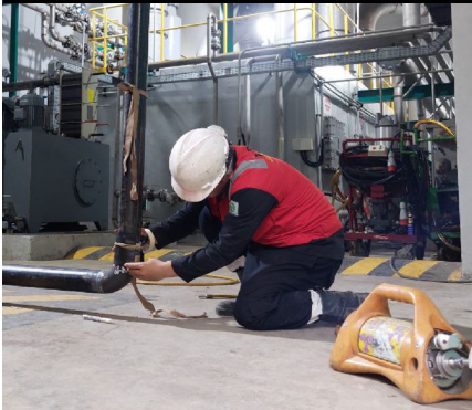
Magnetic Particle Inspection
